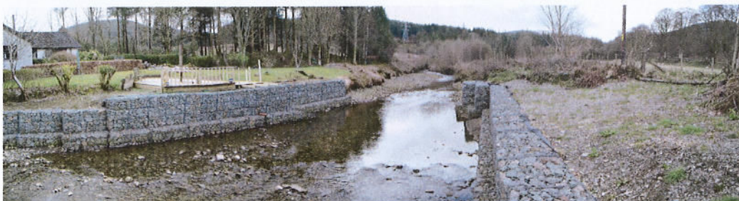
New weir/gauging station area
